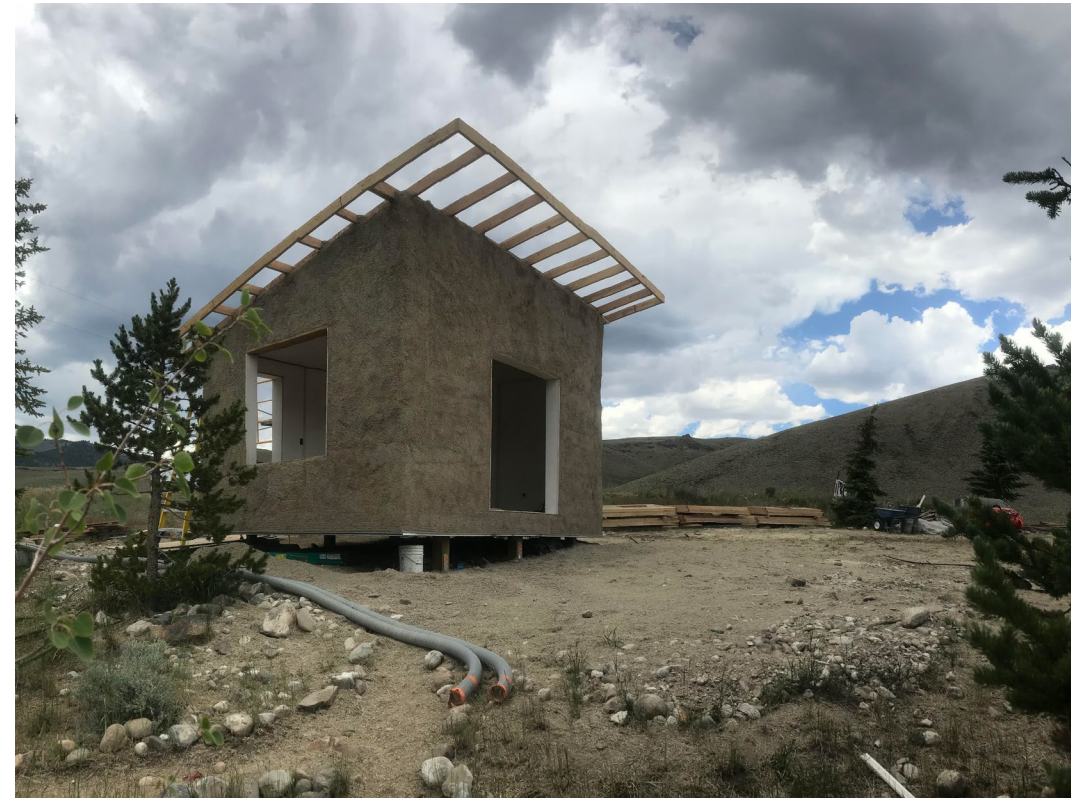
Fig 7.1 Structure using blown hemp+lime
