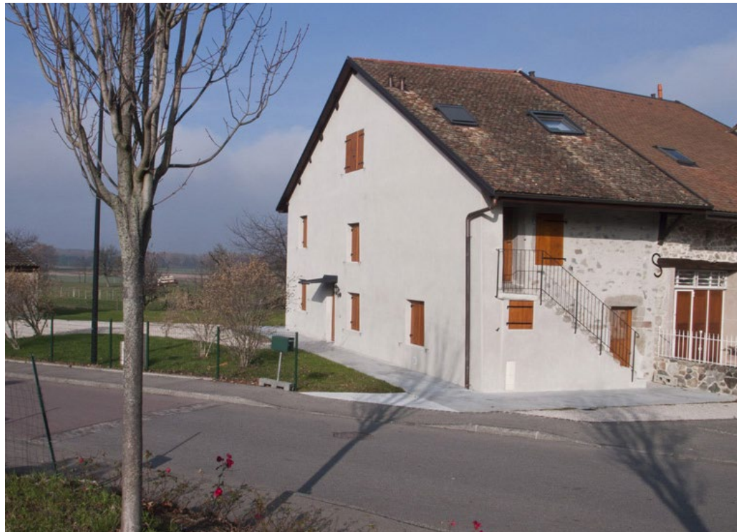
Fig 8.9 Douvaine Renovation by FRAR, Lac Léman, France
