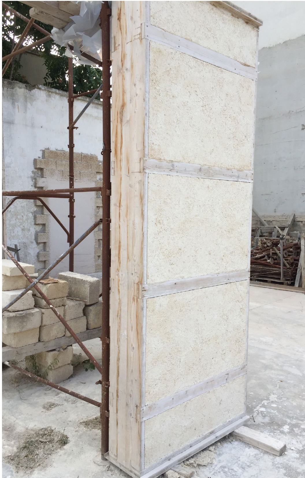
Fig 6.13 Prefabricated hemp+lime wall panels, Puglia, Italy
