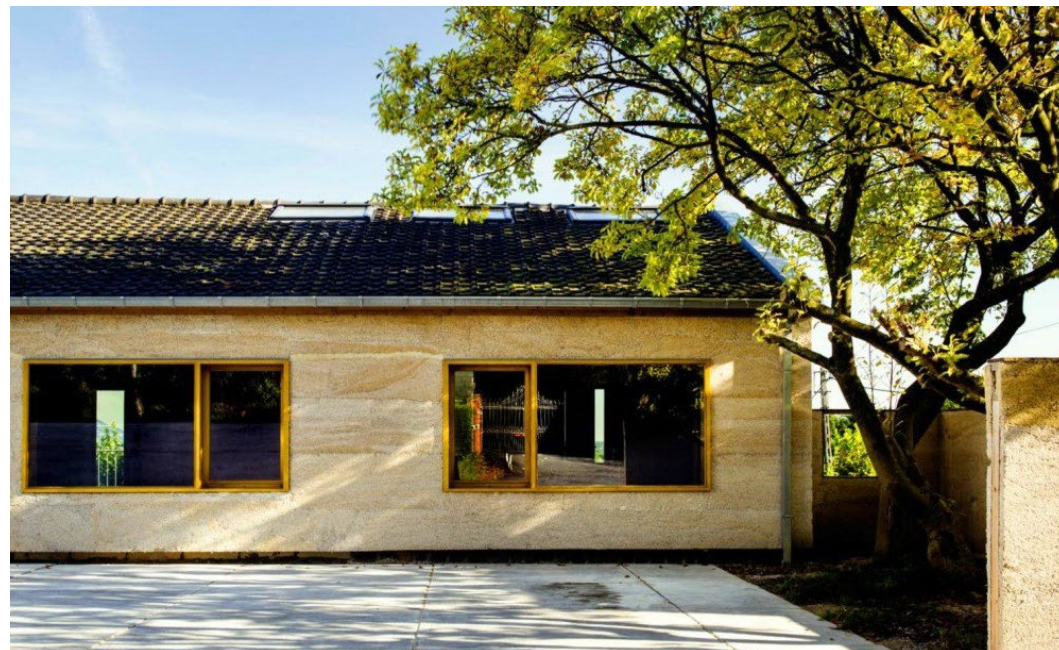
Fig 8.7 Guilleminlan by Martens Van Caimere Architecten, Geraardsbergen, Belgium
