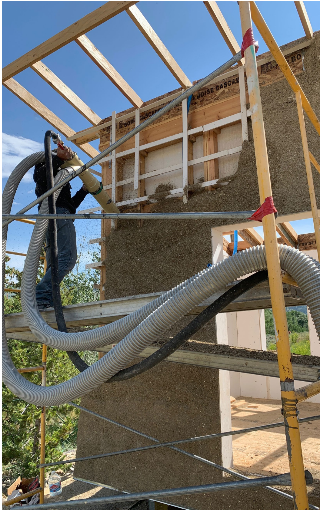
Fig 7.3 Blown system for cast in place hemp+lime construction
