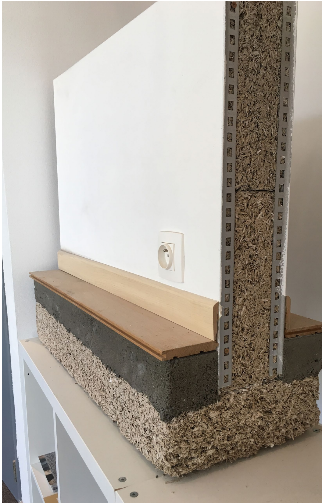
Fig 6.6 Typical hemp+lime interior wall section
