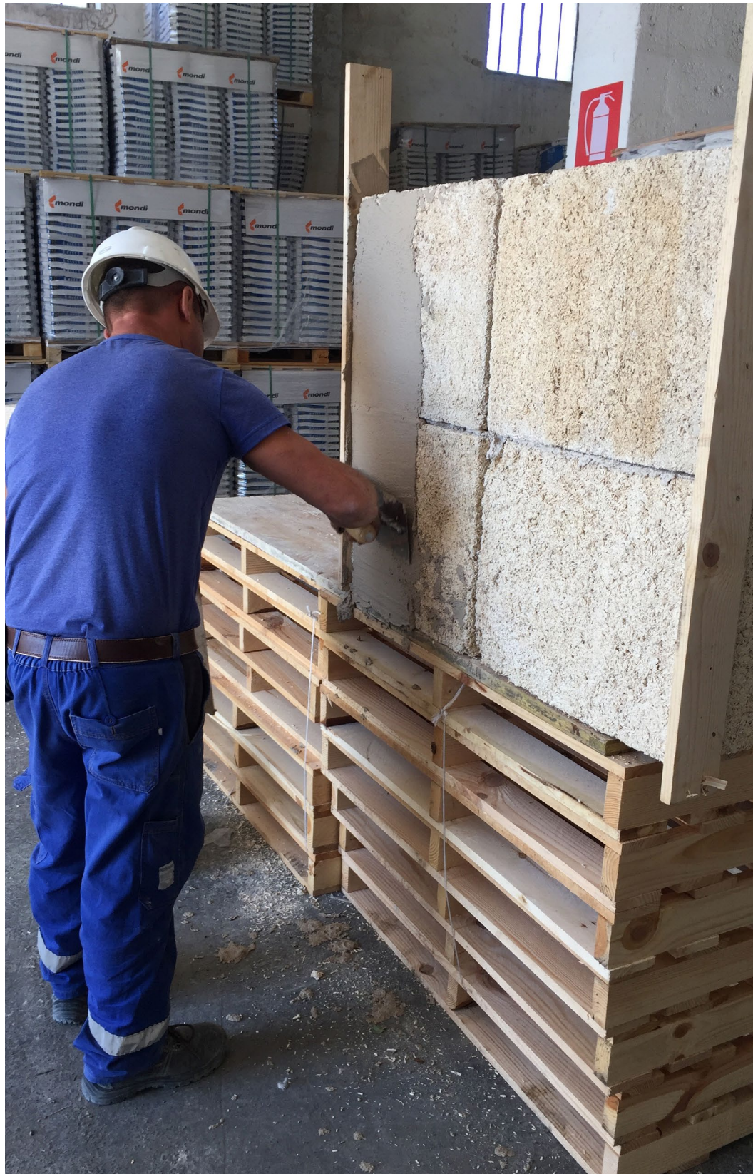
Fig 6.17 Application of hemp and lime plaster
