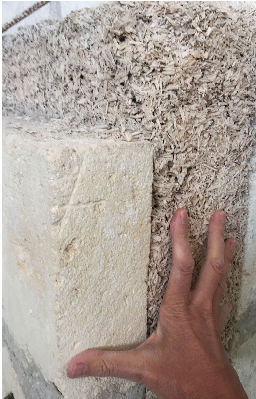
Fig 6.15 Masonry block and hemp and lime insulation
