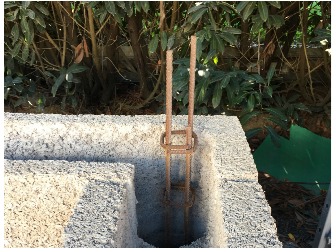
Fig 6.7 Isohemp hemp+lime walls and concrete structure
