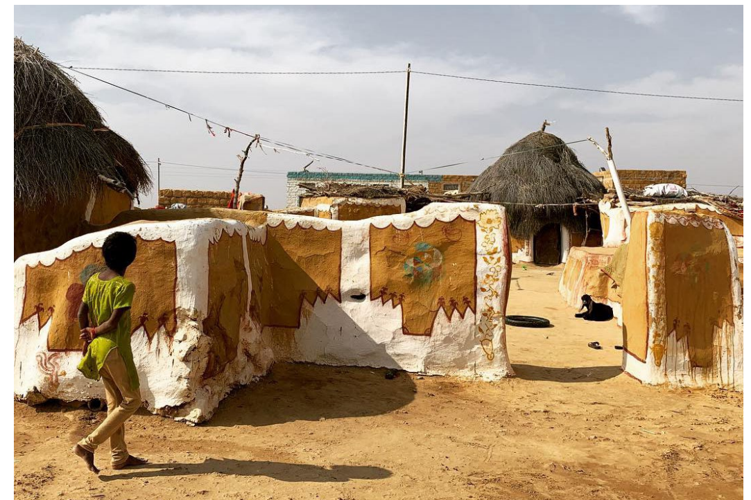
Fig 4.4 Lime paint over cow dung plaster in desert village homes, Jaisalmer, India
